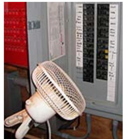
to heat up. An infrared temperature gun is a relatively inexpensive and quick way to spot overheating breakers or other gear. (See "Tools of the Trade" at [www.poultryhouse.com](http://www.poultryhouse.com).) If breakers are hot or are tripping often, we need a qualified electrician to tell us why they are hot and how to fix the problem.
