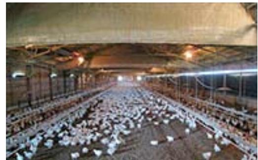
**In high-ceiling houses, air deflector baffles placed lower than about 9 feet above the floor will restrict airflow too much, lowering wind-chill cooling and increasing fan static pressure.**
