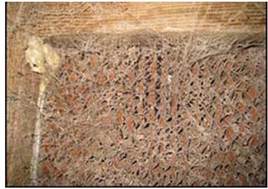
**Insects, dust, dirt, and dander can quickly clog evaporative cooling pads during summer months. Keeping the pads clean greatly improves airflow and bird cooling.**
