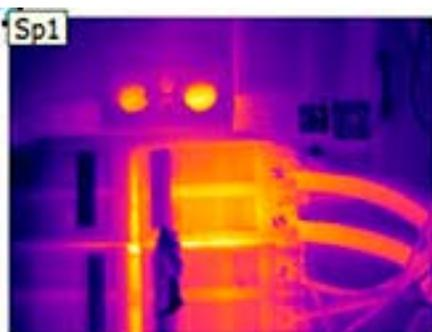
**An overheated breaker like the one shown in the infrared photo at left is big trouble about to happen. Pointing a fan at the breaker box is at best a mere band-aid until the electrician arrives. An infrared temperature gun is a relatively inexpensive and quick way to spot overheating equipment.**
